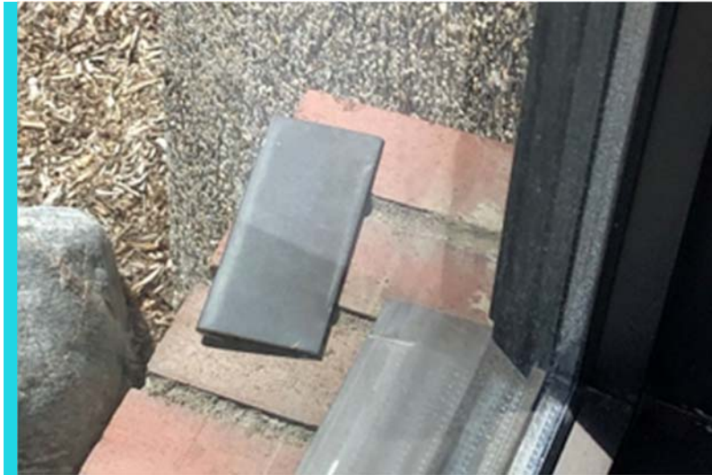
Fig. 49 - Exterior Windows Source: Dialog
