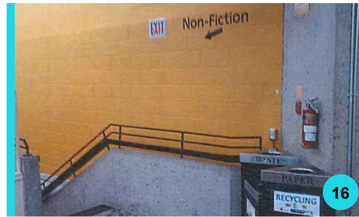
Fig. 108 - Stairs from Upper Level to Study/Non-Fiction – Upper Level Source: RPG
