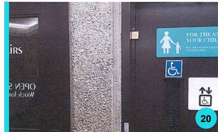
Fig. 112 - South Central Elevator Entrance – Lower Level Source: RPG
