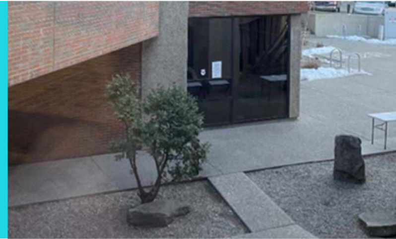
Fig. 87 - South Wing Main Entrance at Lower Level Source: Dialog
