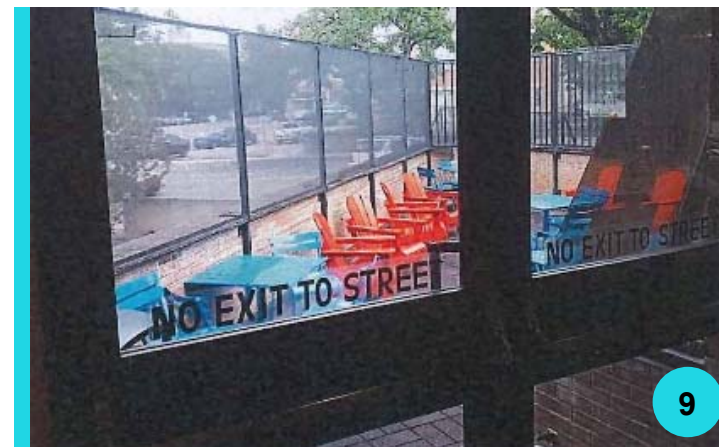
Fig. 101 - View to Patio from Approach to North Stairwell – Upper Level Source: RPG
