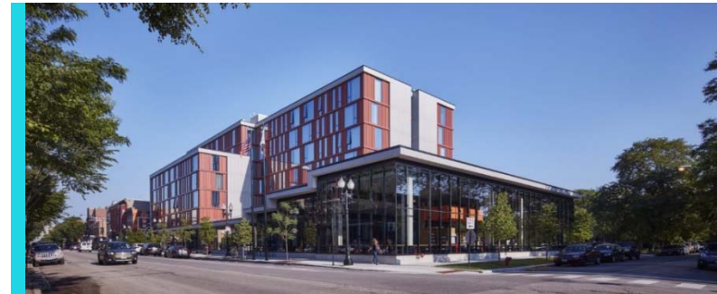
Fig. 28 - Taylor Street Apartments and Chicago Public Library – Little Italy Branch, Chicago IL | SOM
