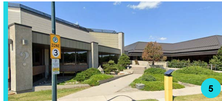
Fig. 97 - Library from Stafford Drive with Receding Windows Source: RPG
