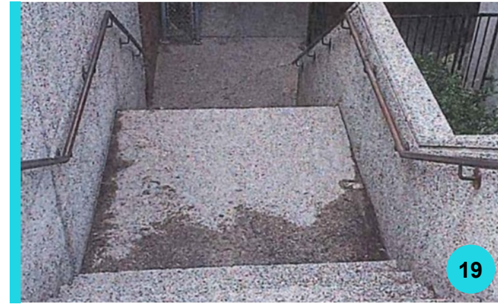
Fig. 111 - Exterior Stairs between North and South Wings Source: RPG
