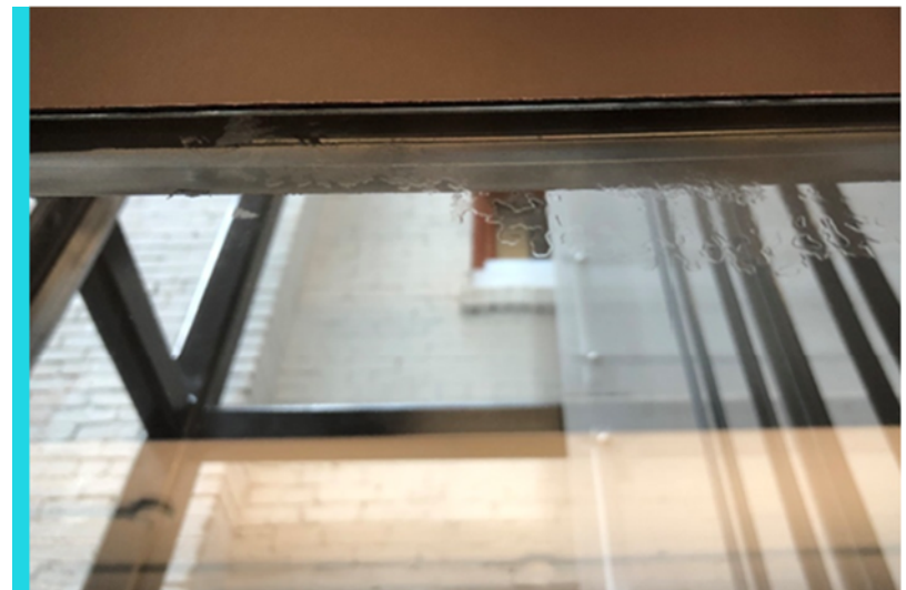
Fig. 48 - Exterior Windows Source: Dialog
