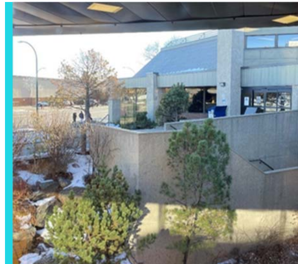
Fig. 90 - Looking South into Millennium Gardens and to Main Entrance Source: Dialog
