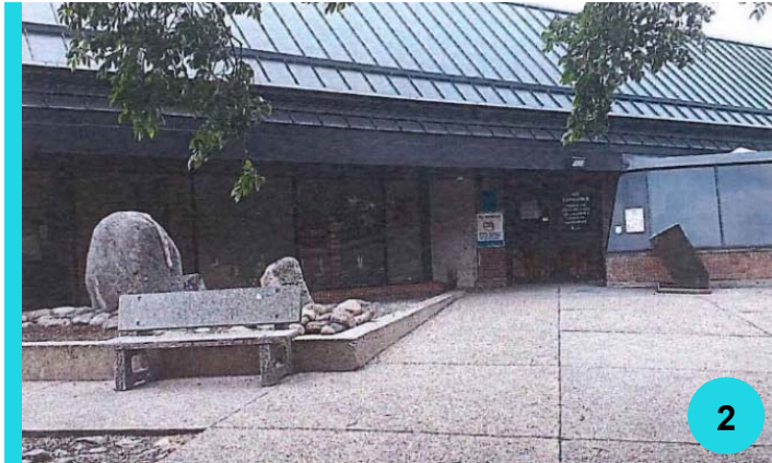
Fig. 94 - View to Doors (no access) to North Wing from Stafford Drive South – Upper Level Source: RPG
