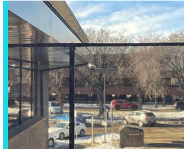
Fig. 89 - North Wing Upper Level Patio West to Parking Area Source: Dialog
