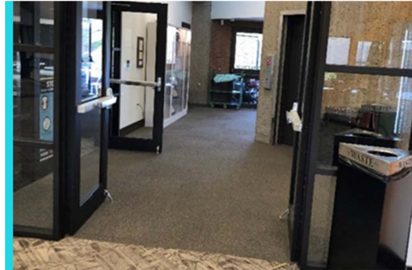
Fig. 64 - North Wing Emergency Exit (elevator, stairs, and patio)
