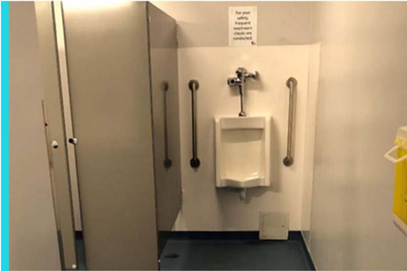
Fig. 66 - North Wing Washroom
